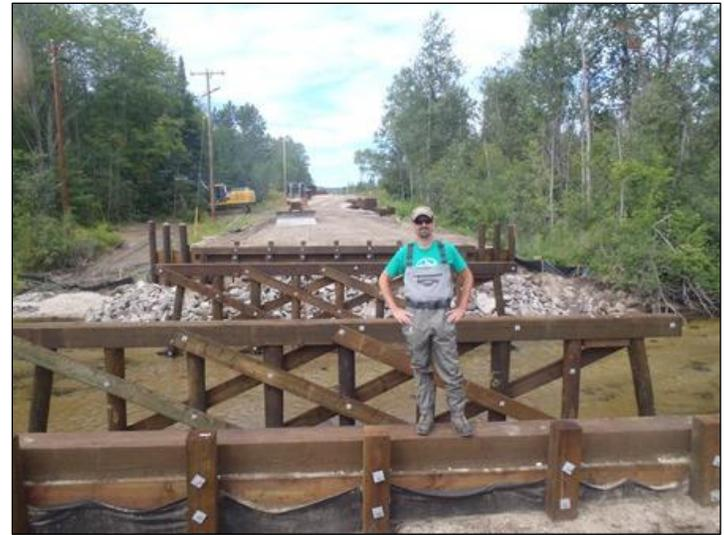
During - Timber piles and abutments were installed
